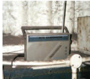
Sprayed coatings on wall
