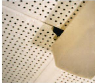
Asbestos insulating board ceiling tiles
