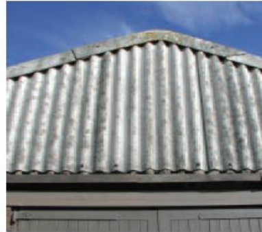
Asbestos cement panels
