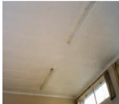
Asbestos insulating board panels
